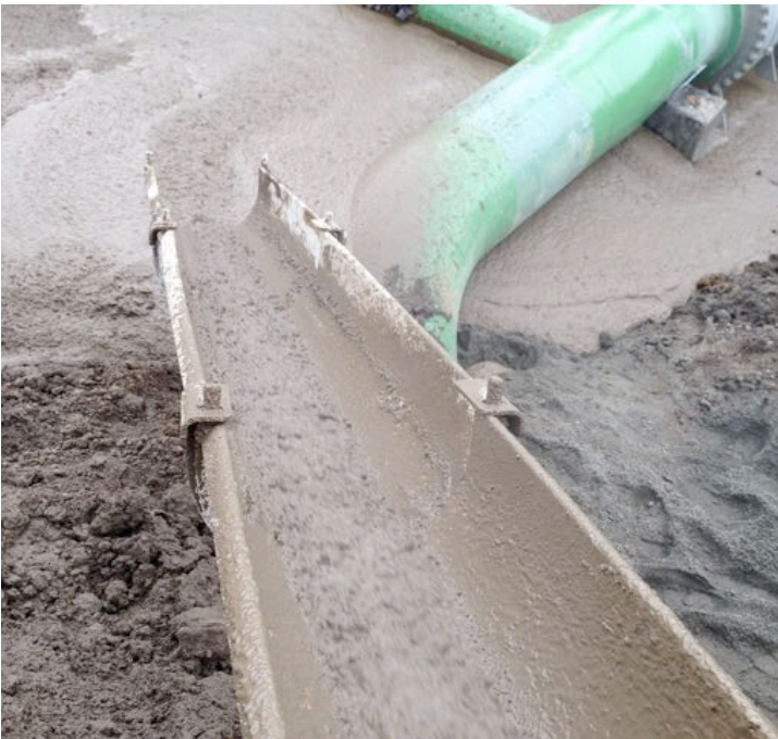
Figure 4 Fresh Flowable Fill
