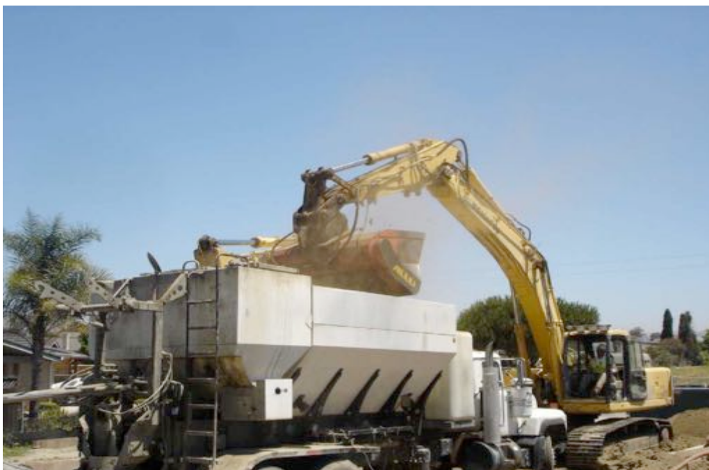
Figure 6 Allu Shredder on Excavator Loading Soil Hopper on Volumetric Mixer
