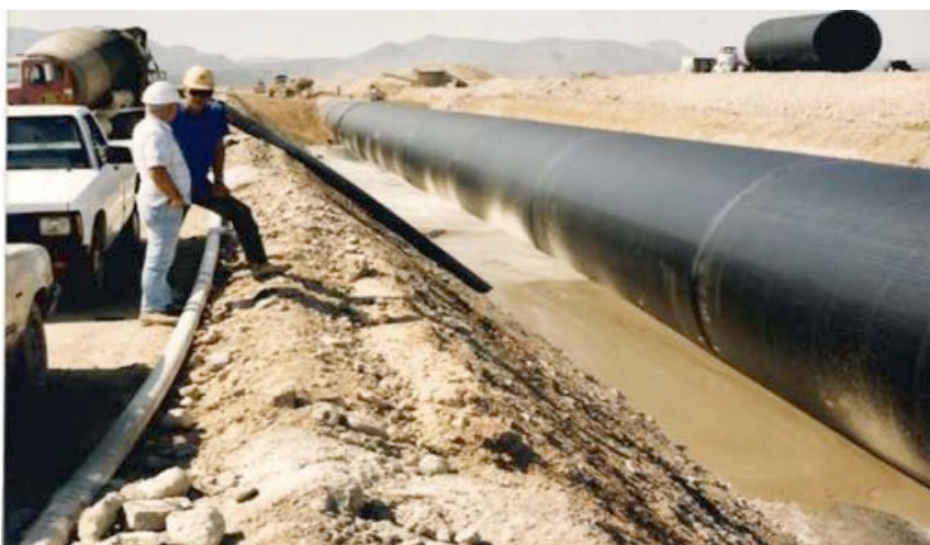
Figure 8 Flowable Fill on the CAP 21-ft Steel Pipe
