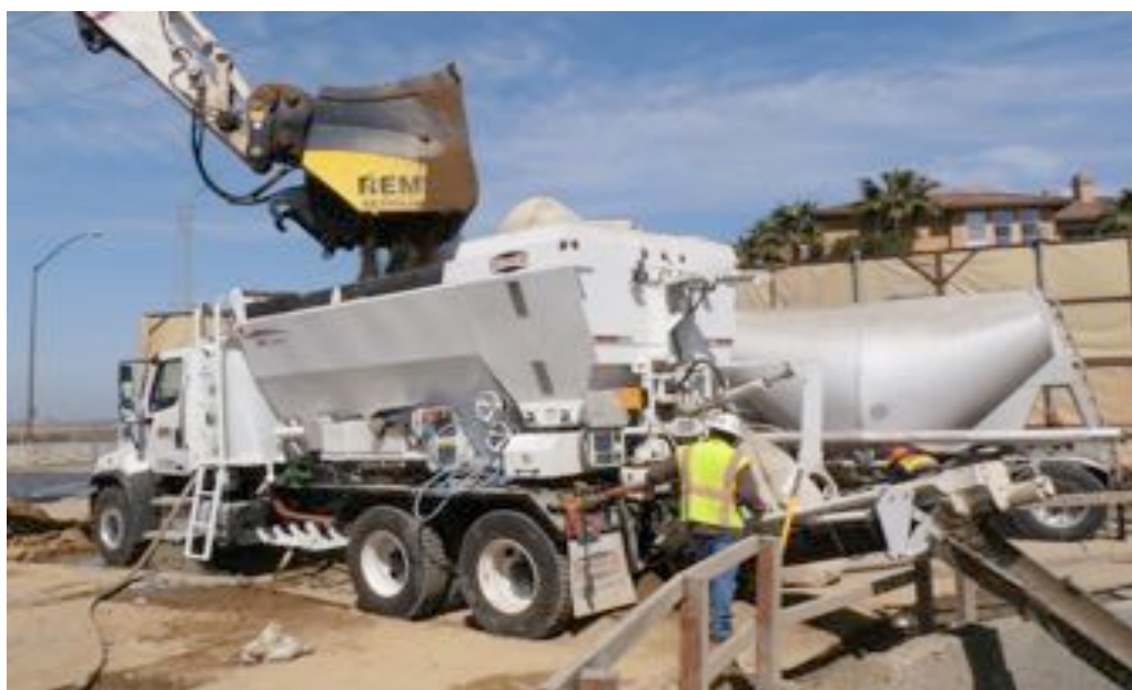
Figure 6 Remu Shredder bucket on excavator loading material
