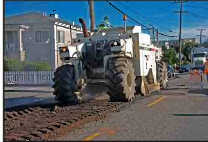
2. PULVERIZE DETERIORATED PAVEMENT
