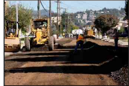
3. RESHAPE FOR NEW HMA OVERLAY
