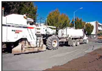
5. MIX – HYDRATE CEMENT & RECYCLED BASE
